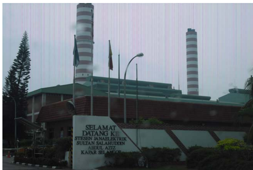
Figure 1.2: Salahuddin Abdul Aziz Shah power plant in Kapar Selangor.
