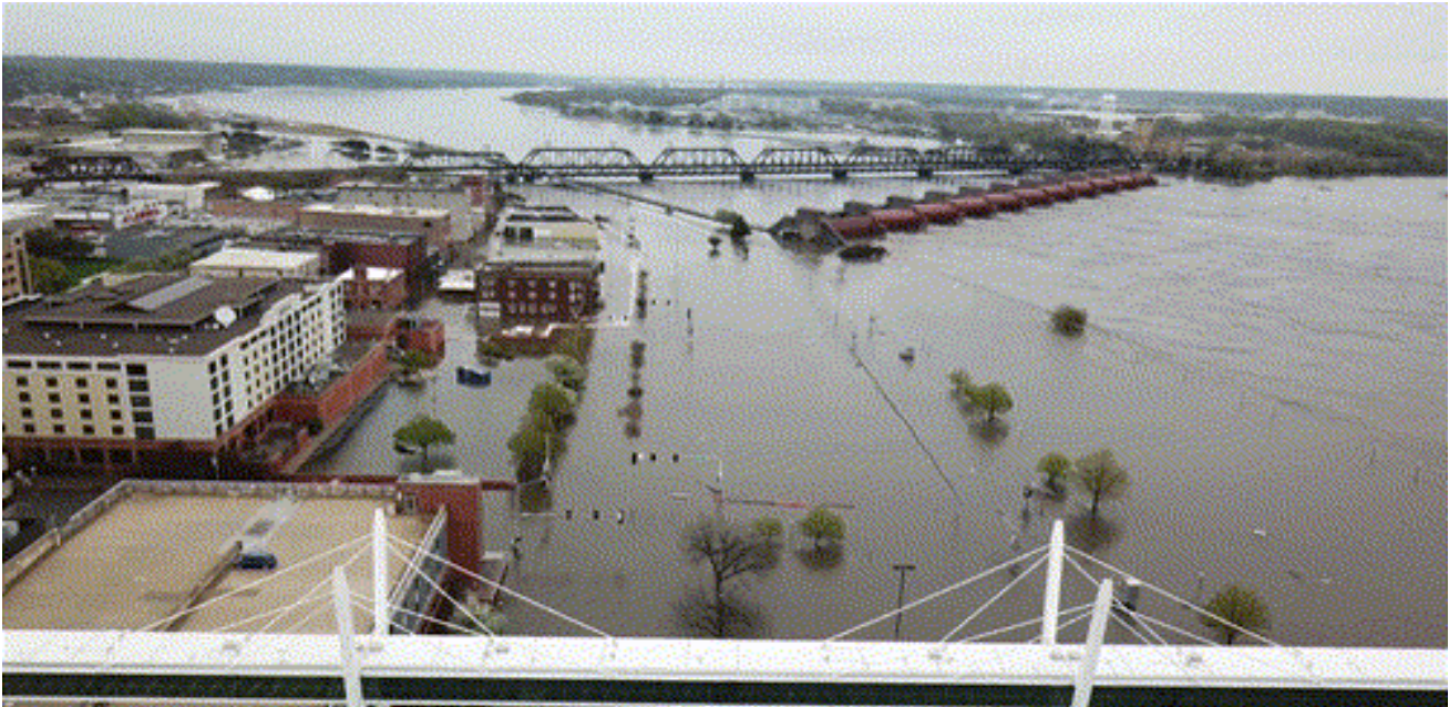
Figure 1.3: River/Fluvial flood (Davenport, Iowa 2019)
