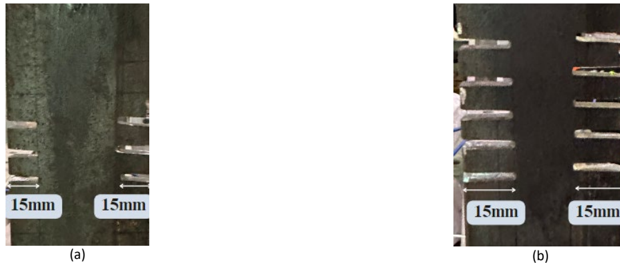
Figure 3 Damage on the structure (a) 3 cuts with a depth of 15 mm (b) 5 cuts with a depth of 15 mm
