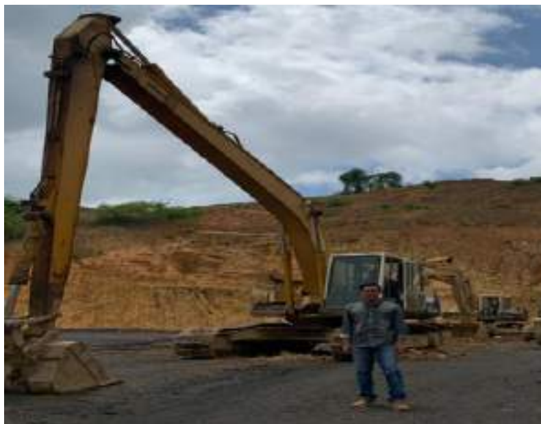
Figure 5: Site Photography showing Hydraulic Excavator 350 Komatsu
