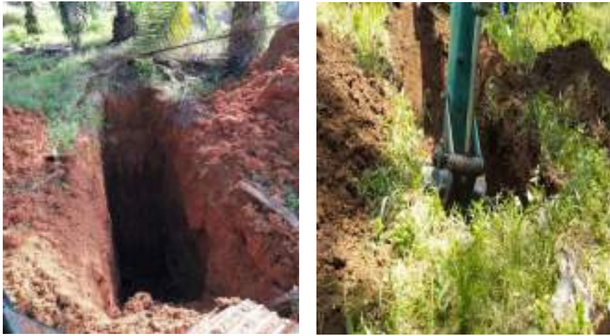
Figure 6: Site Photography showing trial pit at site
