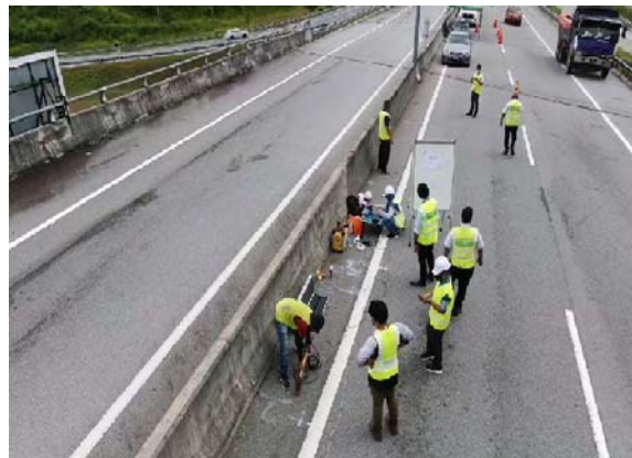
Figure 6b. Demarcation of excitation points and accelerometers location
