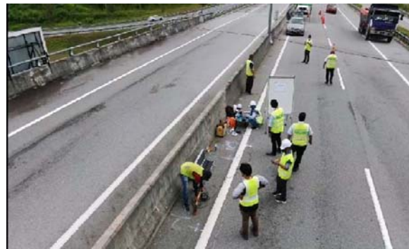
Figure 12. Hammering points is in progress to get bridge response in term of frequency and mode shapes.
