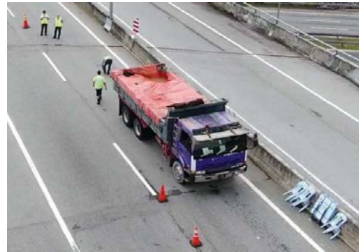
Figure 13b. OMA test on the RC bridge deck in progress.
