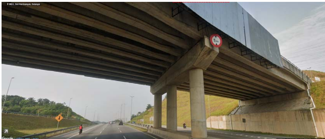
Figure 10. Physical view of bridge underneath.
