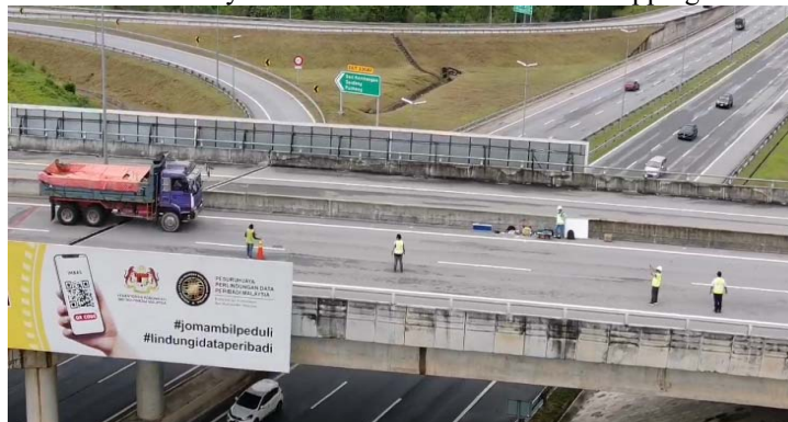
Figure 20a. Force vibration test (Operational Modal Analysis-OMA).
