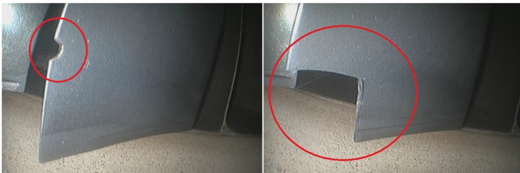
Figure 1.2 Multiple instances of blade damage found during the periodic and borescope inspections of the gas turbine
