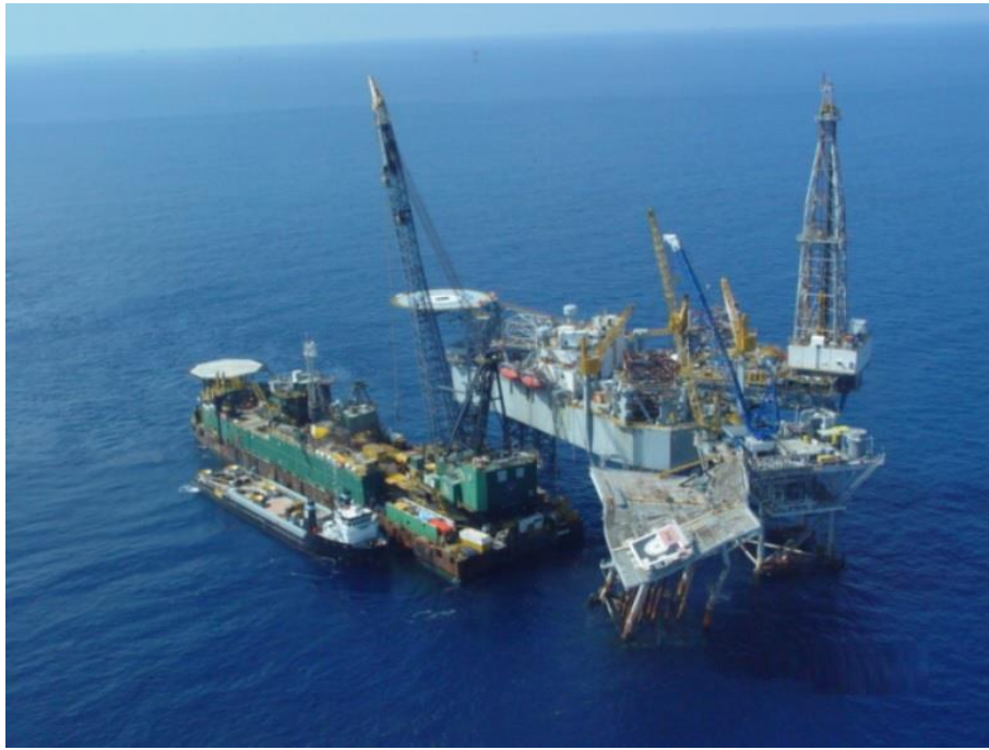
Figure 1.2 EI-322 'A' platform structures damaged by Hurricane Lilli Source: (DeFranco et al. , 2004)
