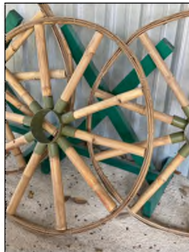
Middle-size Radial Ring of Bamboo Pavilion Source: Meor Razali et al 2022
