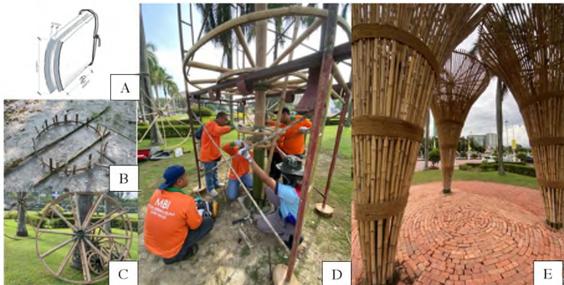
Figure 7. Construction of Bamboo Pavilion.
