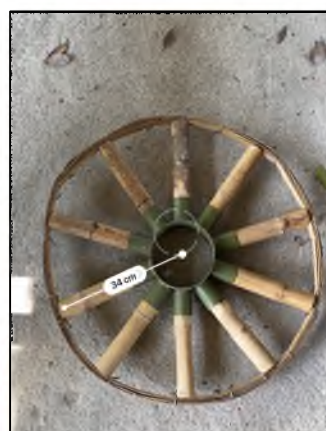
Small-size Radial Ring of Bamboo Pavilion Source: Meor Razali et al 2022
