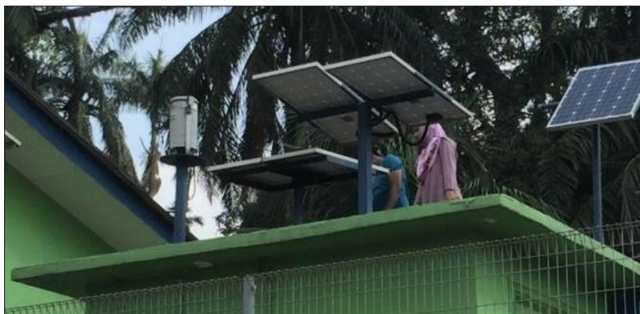
Figure 4. Tipping Bucket installation at the top of the station housing [16]
