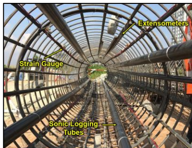
Figure 6. Test pile instrumentation
