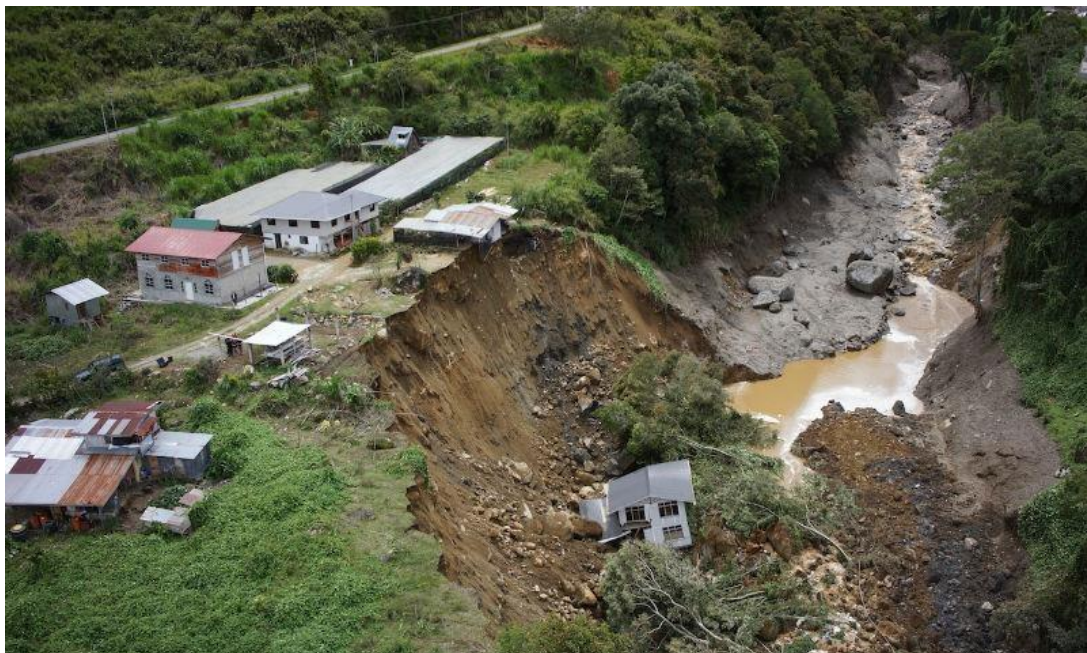
Figure 1.8 The collapse of homestay into the Mesilau river due to the earthquake induced landslides ( source from NST, 2015; The Star, 2015 ).
