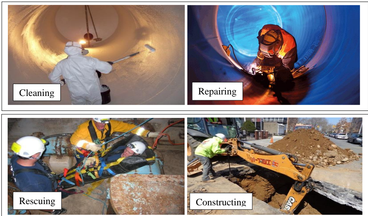
Figure 1.2 Activities in confined space
