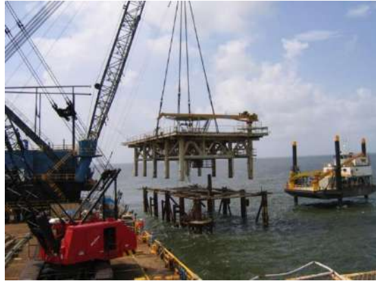
Fig. 1 Decommission of obsolete offshore structure (BSEE 2016)
