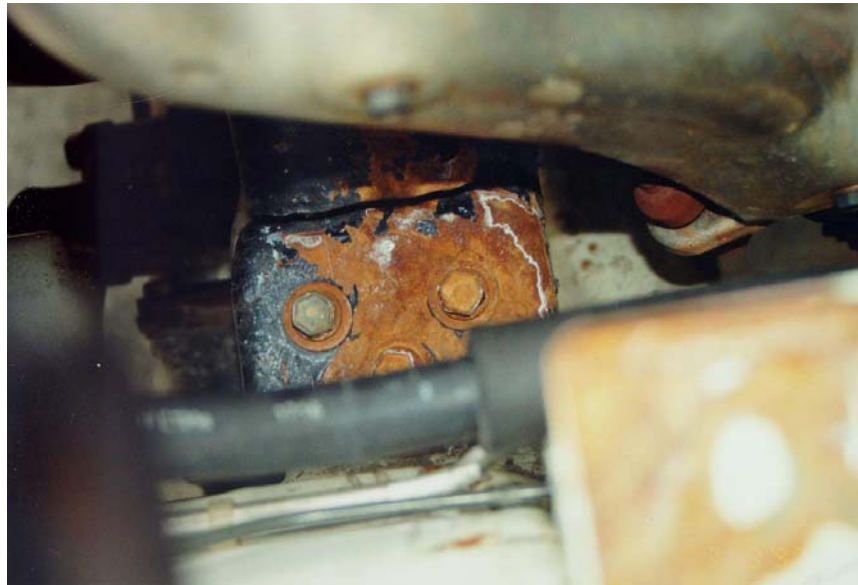
Figure 3: Battery acid discharged to the vehicle chassis
