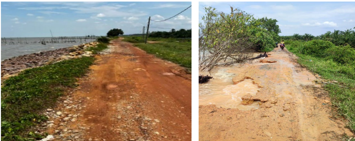
Fig. 7 - Coastal bund without mangrove ecosystem before and after high tides phenomenon
