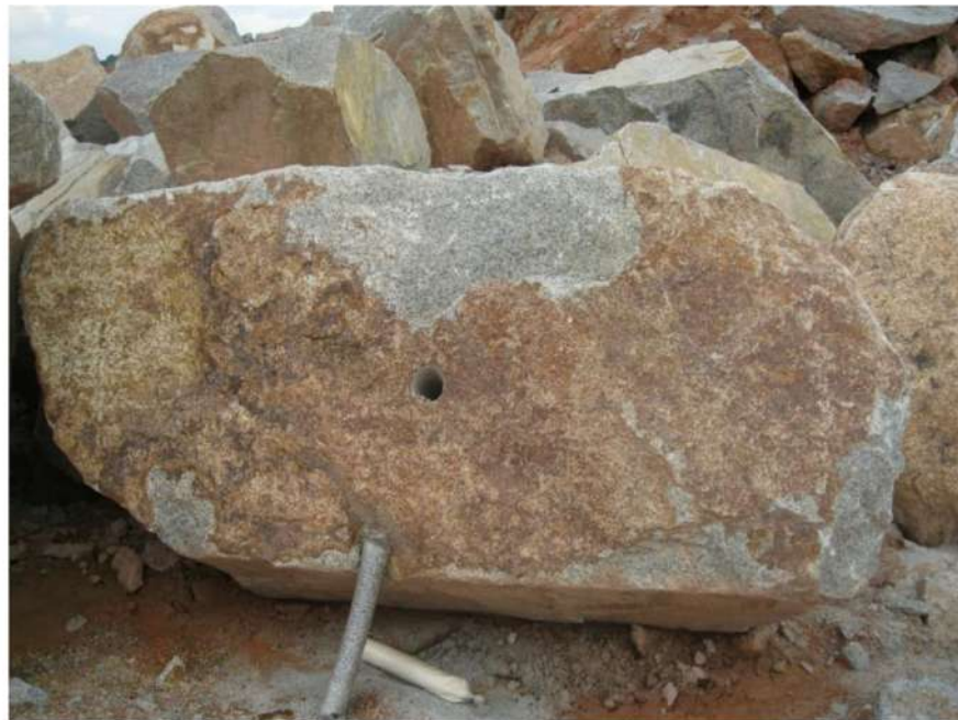
Figure 9. The drilled hole in the oversize boulder for charging and blasting operation.
