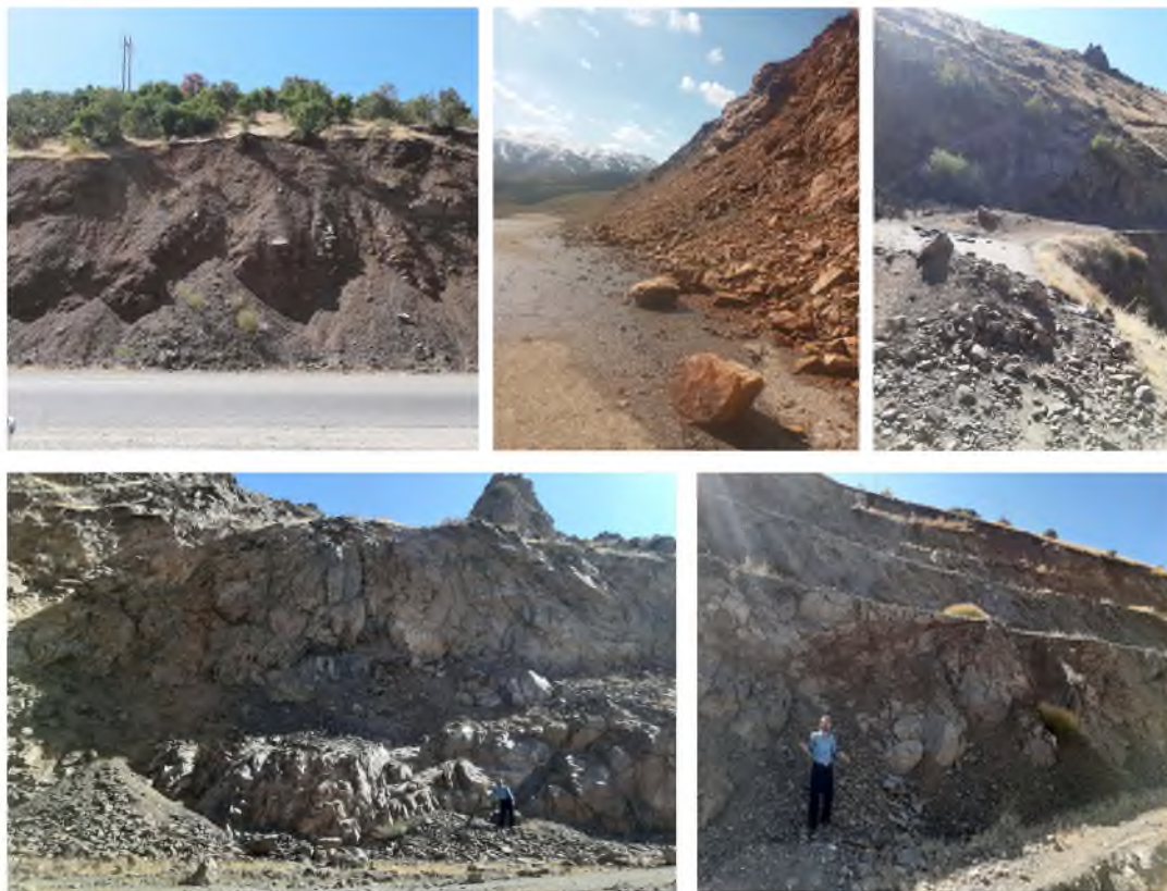
Figure 2. Different types of landslides observed along the Saqqez-Marivan road in the Kurdistan Province of Iran.
