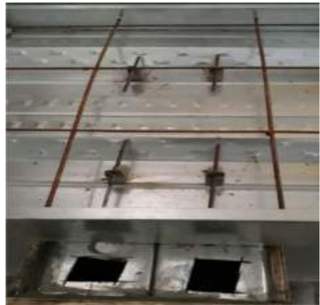
Fig. 24 Brackets “fixed by screw” shear connection system
