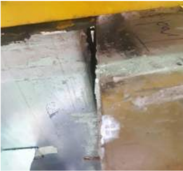
Fig. 50 Transverse slip at the maximum strength capacity of the specimen
