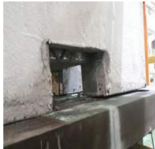
Fig. 41 Failure mode of the toe-to-toe without holes system
