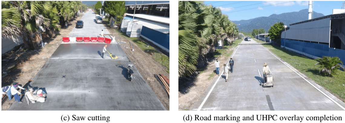
Fig. 10 Pilot UHPC overlay procedure (continued)
