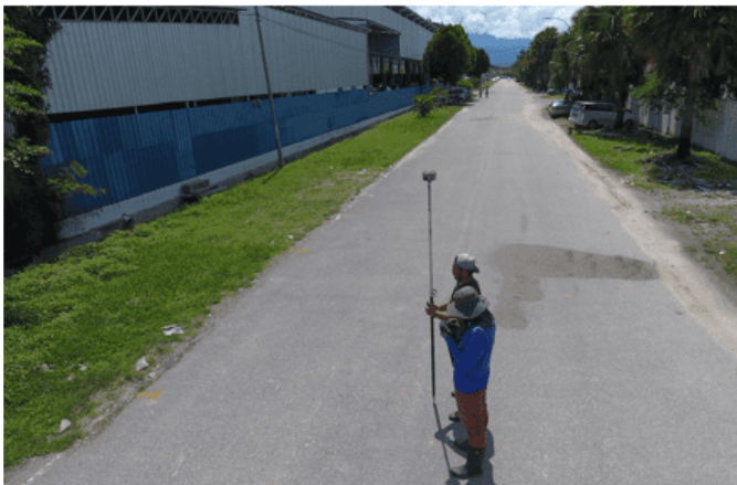
(a) Survey before milling
