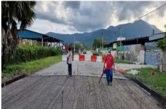
(a) Surface cleaning
