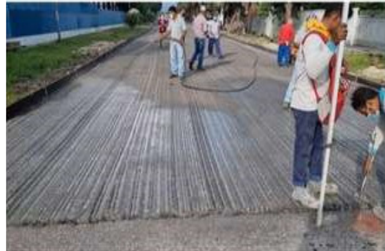
(b) Applying bonding agent
