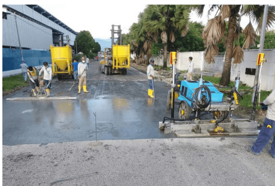
(a) Screeding and leveling
