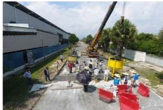
(b) Mobile crane
