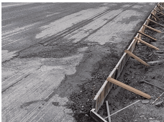
(c) Formwork installation
