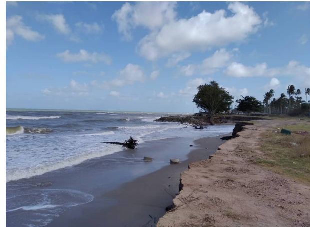
Figure 1 Erosion site at the test area
