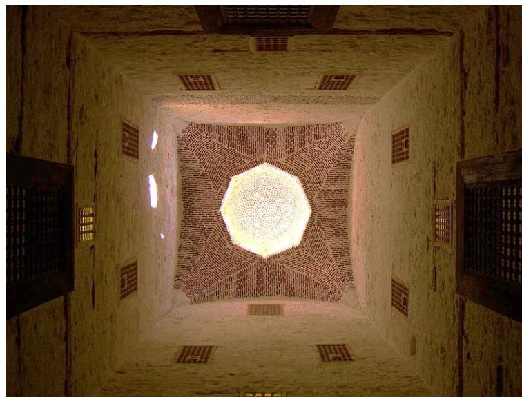
Figure 1 Light well ceiling in Qaitbay Citadel in Alexandria
