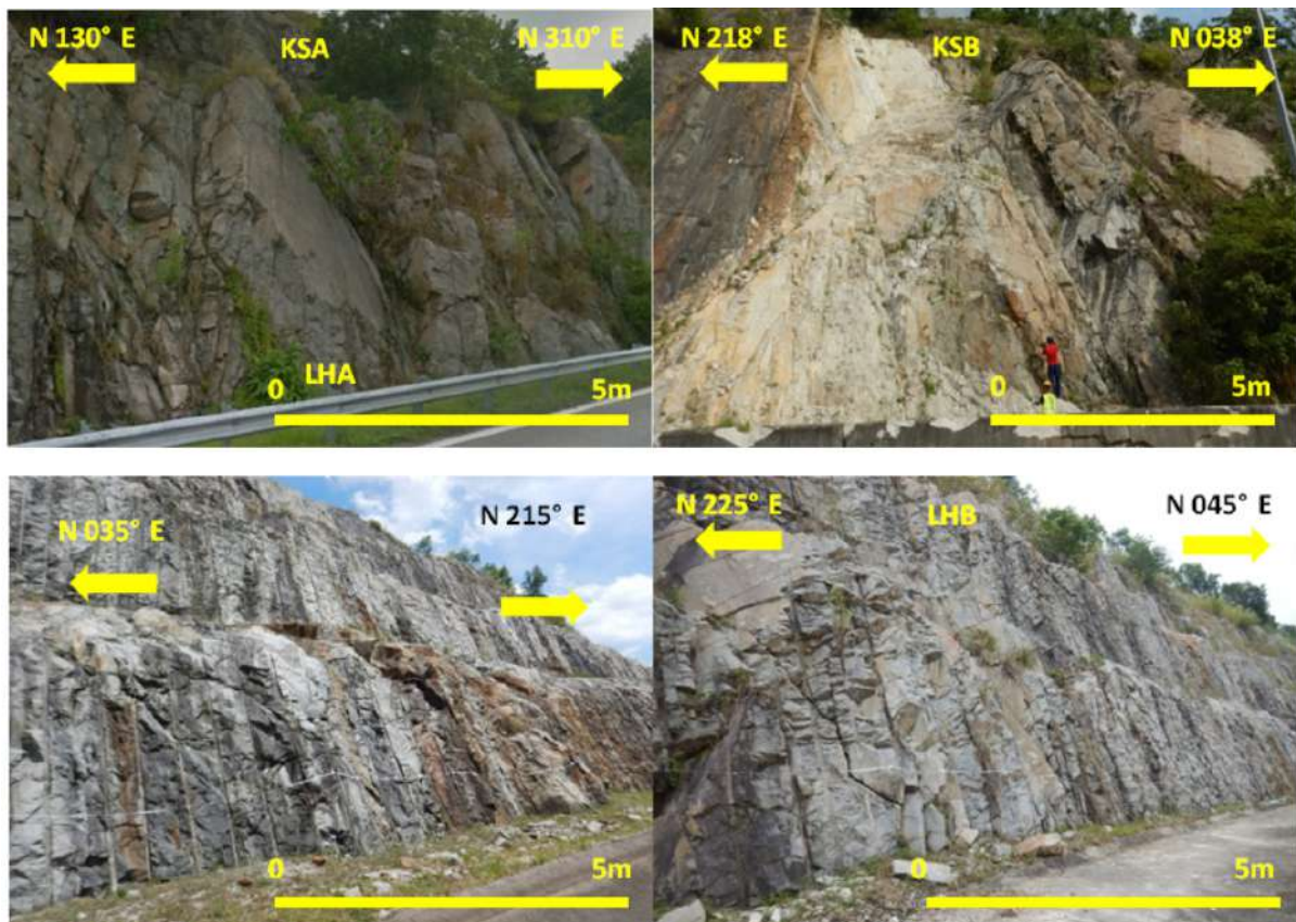
FIGURE 5. Field photo for Slope KSA, KSB, LHA, and LHB. All slopes studied were granite rock cut slopes
