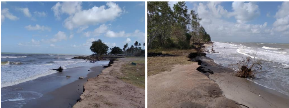
Figure 1. Erosion site at the study area.
