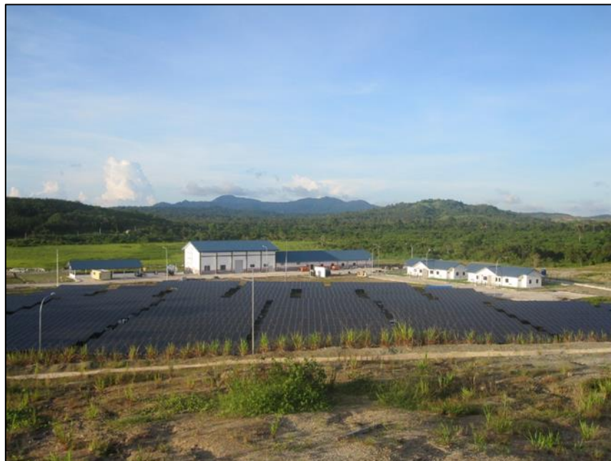
Figure 1.2 View of SHS Pulau Banggi
