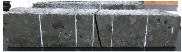
Figure 5 Flexural failure of the tested specimen
