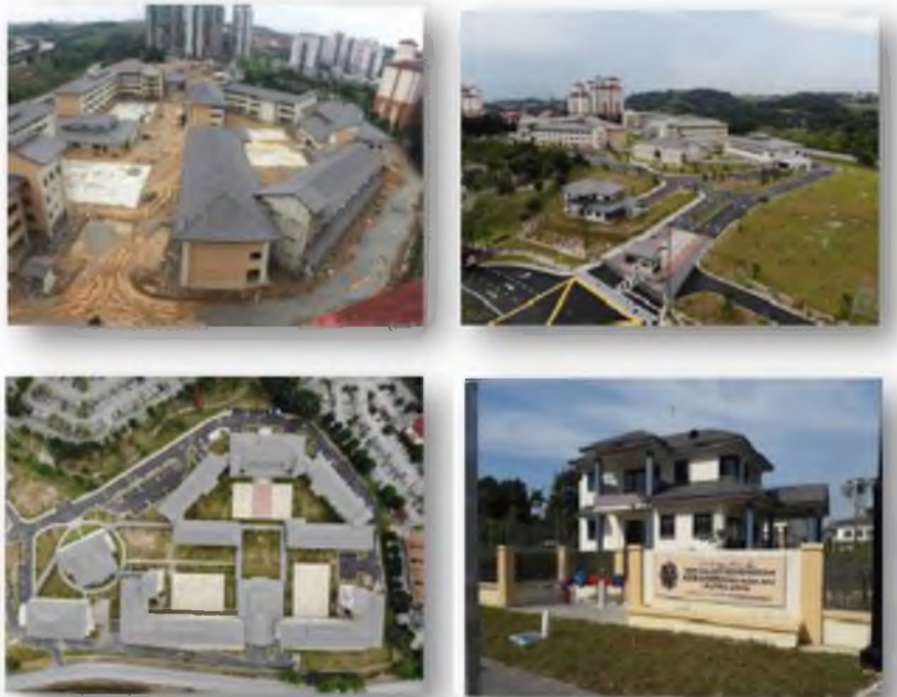
Figure 1.5 Completed project 2018 at SMKA Putrajaya, Presint 11
