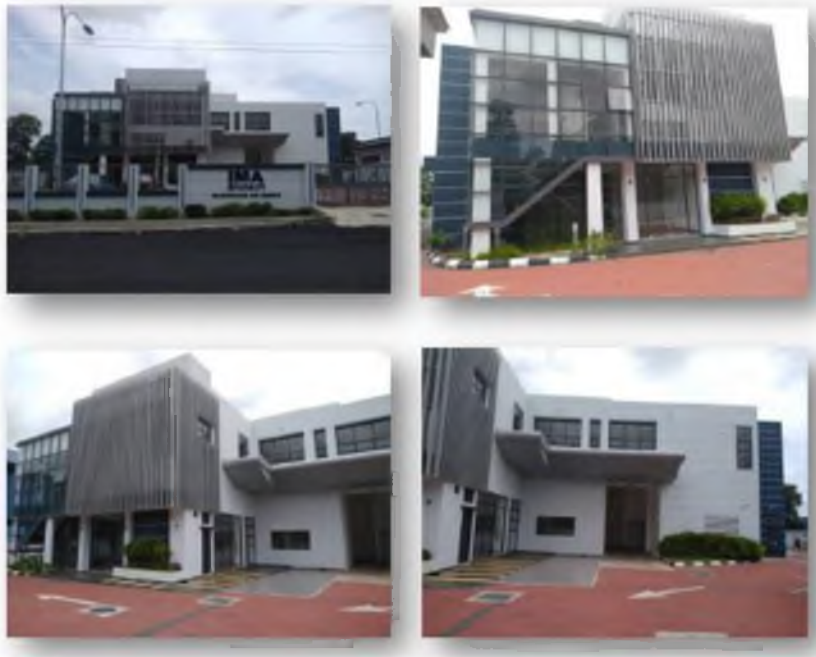
Figure 1.4 Completed project 2017 at Pharmaceutical Factory, Nilai
