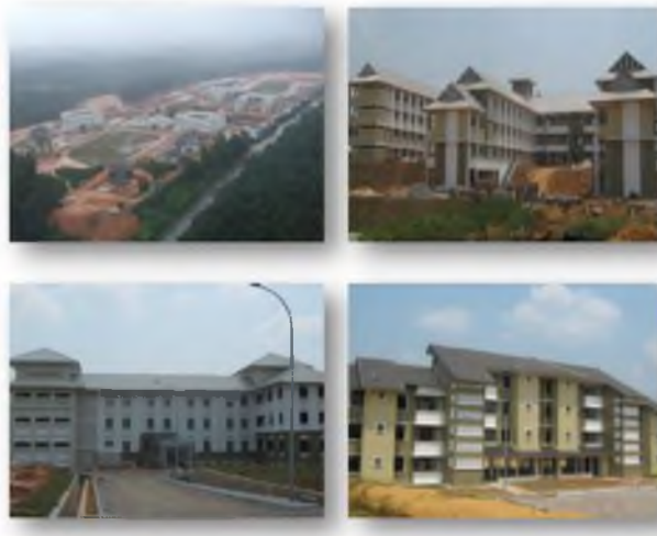
Figure 1.2 Completed project 2011 at Sek. Mek. Sains Semborong, Kluang
