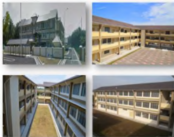
Figure 1.3 Completed project 2014 at Sek. Mek. Keb. Seri Bandar Pontian
