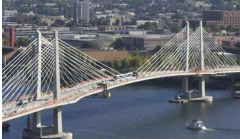
Figure 1.7 Cable Stayed Bridge
