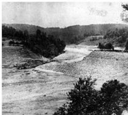
(a) Banqiao Dam (1975)
