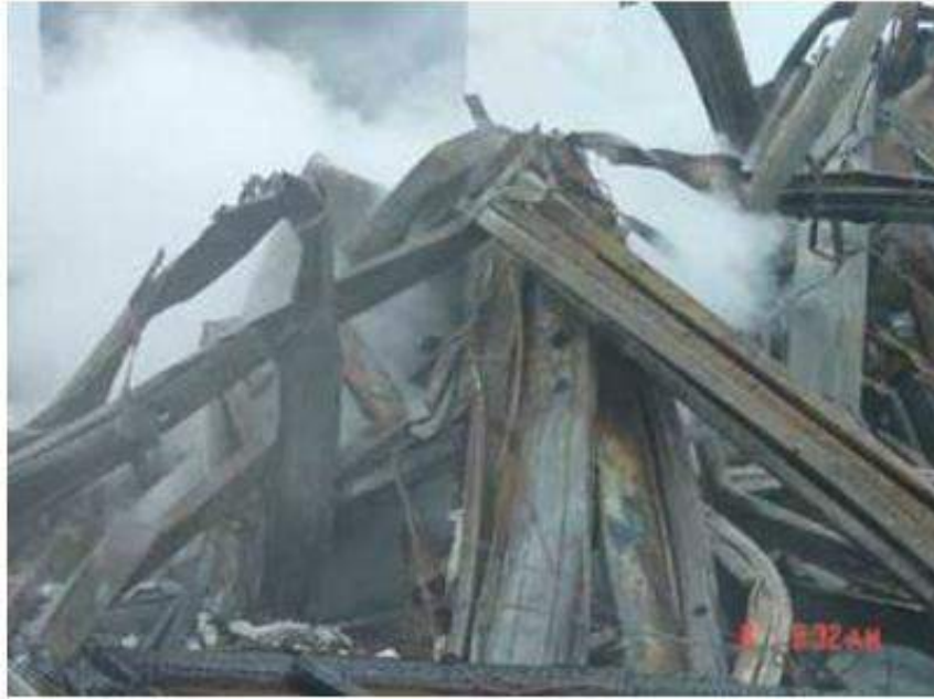
Figure 1.2 Remaining of a lightweight steel frame after a fire (Karl K. Thompson, 2006).
