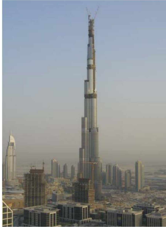
Figure 1.1 Super high-rise building, Burj Khalifa, Dubai constructed using SCC material (Baker et al. , 2009)
