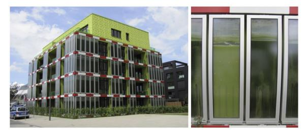
Figure 4 MA-BRF in BIQ house, Hamburg Germany, zoomed image of PBR panels being used as façade (Biloria and Thakkar, 2020).
