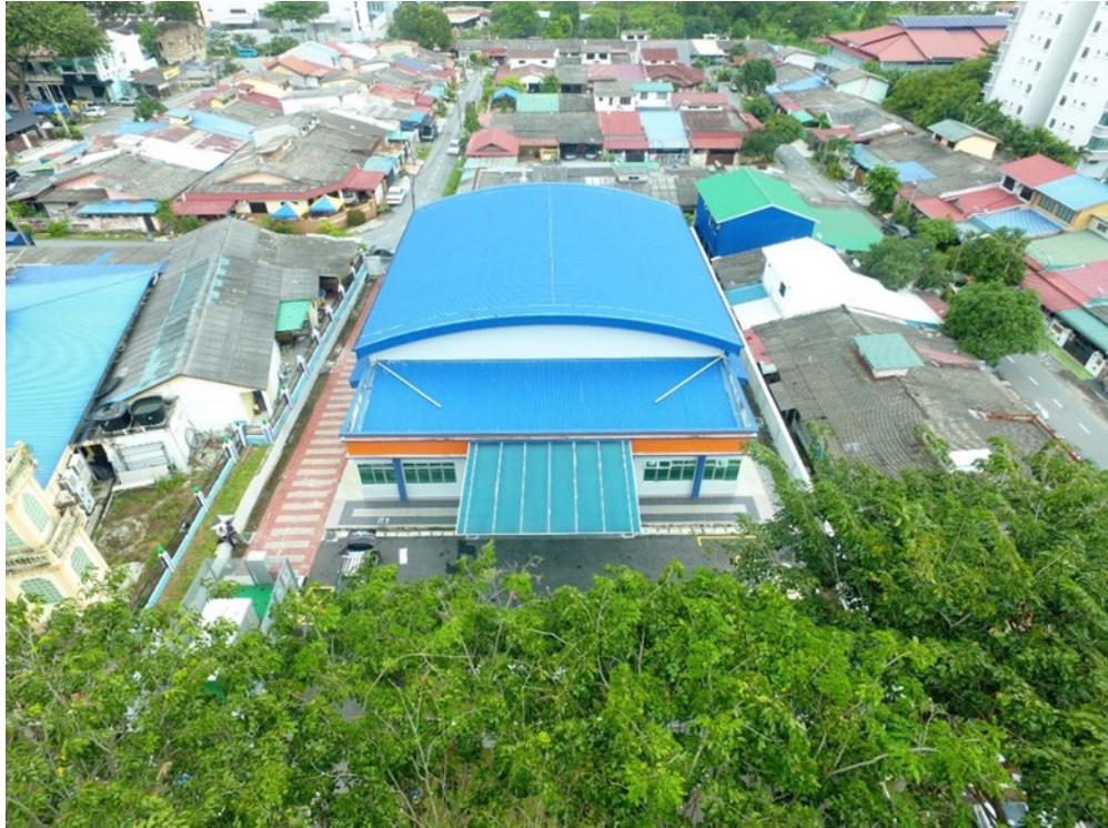
Figure 1.1 Aerial view of Dewan Muafakat Johor Taman Kobena, Tampoi, Johor Bahru. Image taken from a DJI Phantom 4 unmanned aerial vehicle (UAV) from an approximate 35m flight height.
